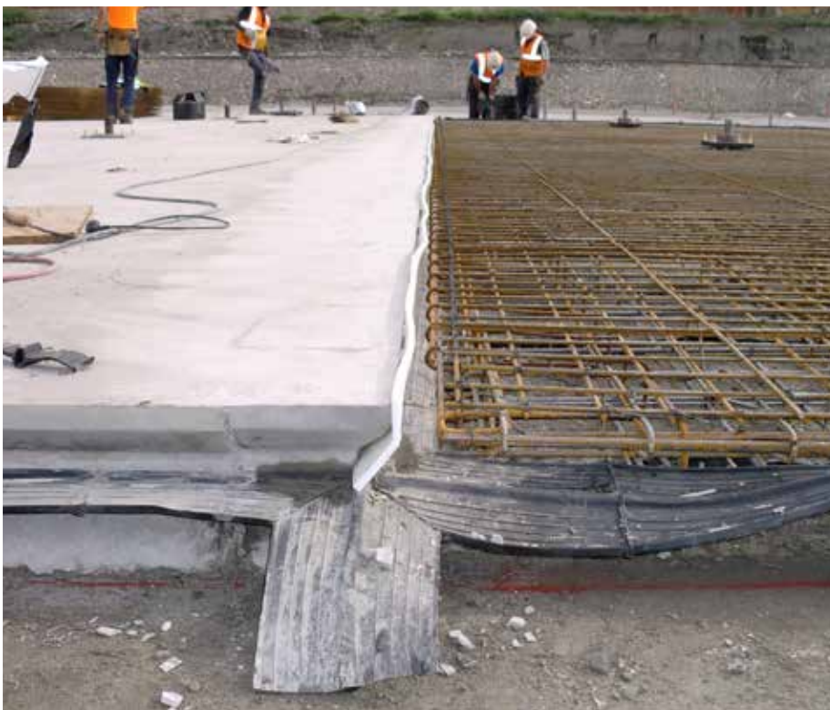
Use of a WATERSTOP BFO profile in a horizontal concrete casting
