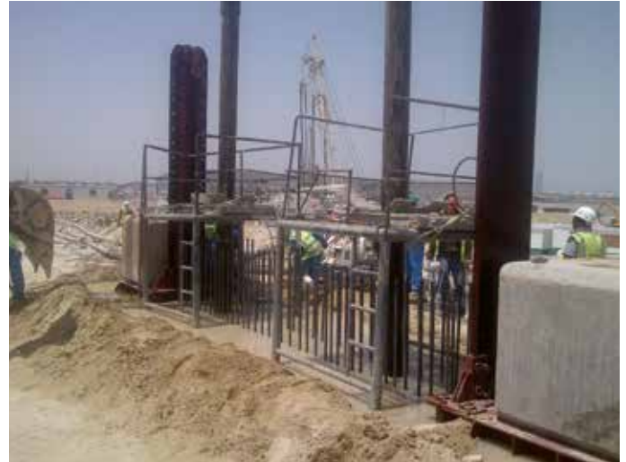
Realization of a diaphragm wall with Waterstop joint
