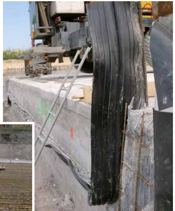
Application of WATERSTOP BFO joint
