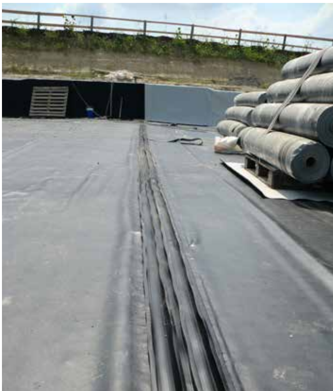
Laying of a compartmental joint welded to a PVC membrane
