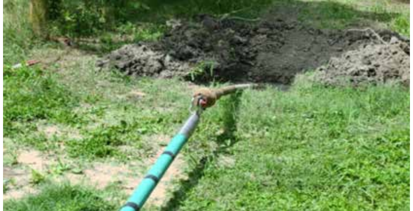
"No-Dig" horizontal injections
