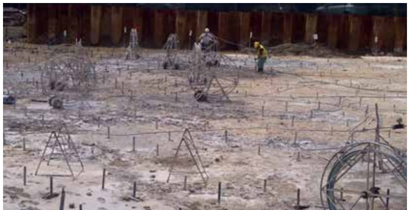
Consolidation grouting
