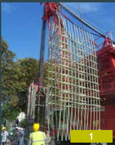
DURGLASS® cage lifting
