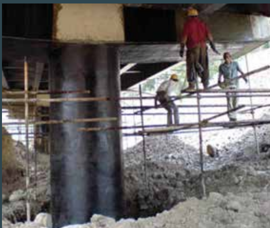
Column reinforcement by means of CARBOPREE® fabric
