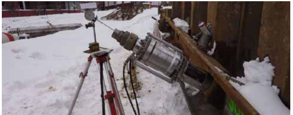
Stretching of a DURGLASS® anchor
