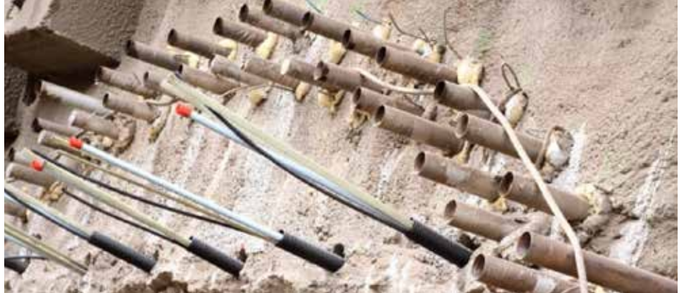
Portal with DURGLASS® glass fiber bolts
