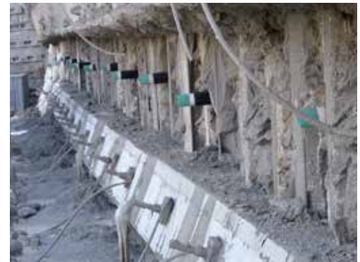
Drains on bulkhead reinforcement
