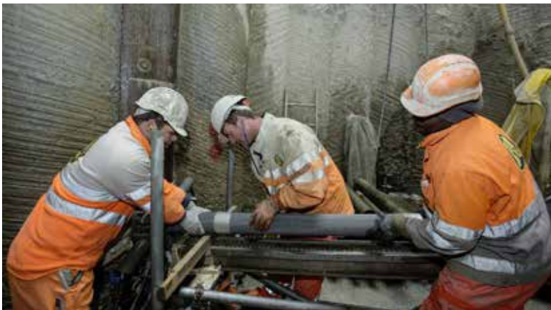
Installation of DWS double wall drain
