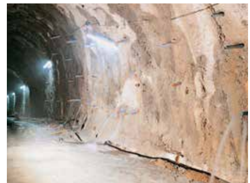
Drains on tunnel masonry vertical structure
