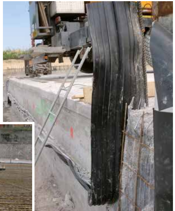
Application of WATERSTOP BFO joint
