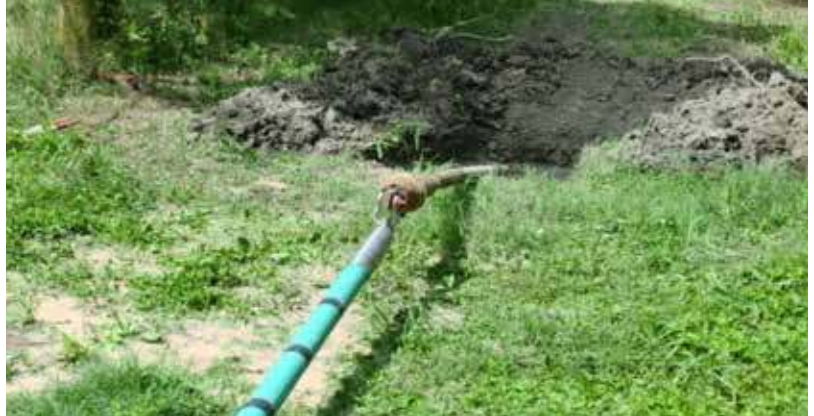
“No-Dig” horizontal injections
