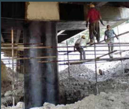
Column reinforcement by means of CARBOPREE® fabric
