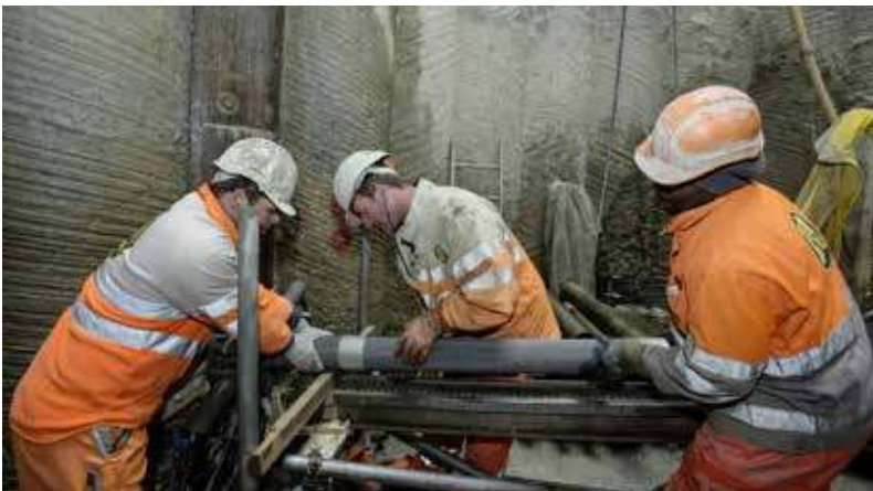
Installation of DWS double wall drain
