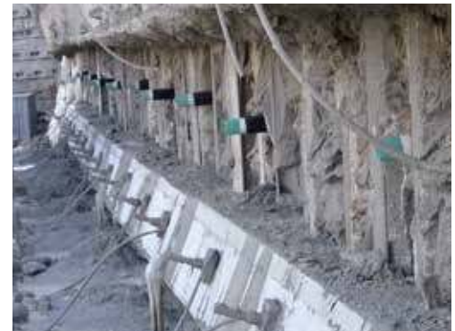
Drains on bulkhead reinforcement
