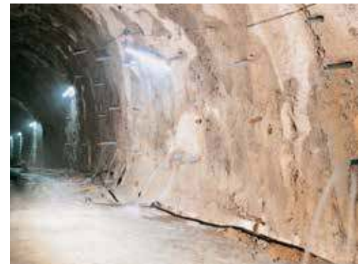
Drains on tunnel masonry vertical structure
