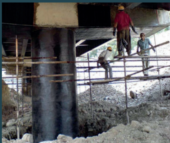
Column reinforcement by means of CARBOPREE® fabric
